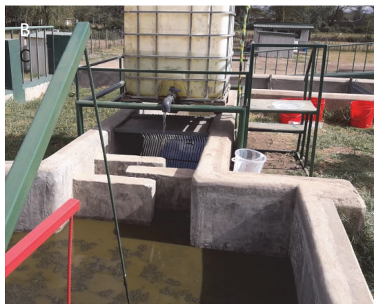
Figure 4.12 A) a Sanivation employee washes detergent, salt, and particulate residue from a geotextile using a high-pressure water rinse and B) example of a conditioner dosing configuration: one dosing port followed by mixing with baffles (photos: Sanivation).
