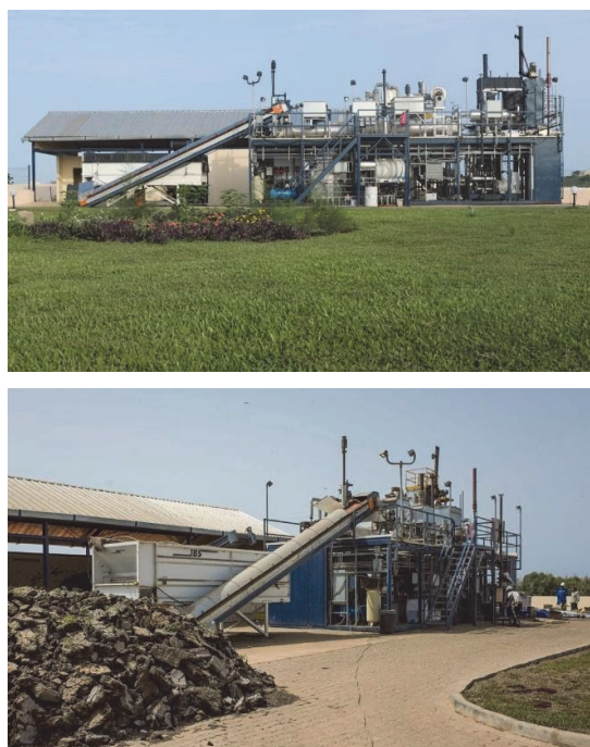
Figure 2.11 The omniprocessor faecal sludge treatment system in operation in Dakar, Senegal (photos: UKZN PRG and Sedron Technologies).
